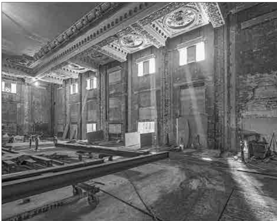
A view of the south wall of the King Street Station main lobby during renovation in the summer of 2012; historic columns are prepped for reinforcement with new steel. John extensively documented the entire King Street Station renovation (including the grand reopening event), and photos are available to view through the Seattle Department of Transportation's Flickr account.
