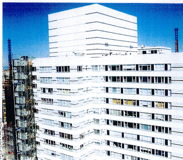
This New York rental property recently underwent recladding. Its former facade had so much water infiltration that the glazed white brick faces popped off. The retrofit improves aesthetics and performance.
