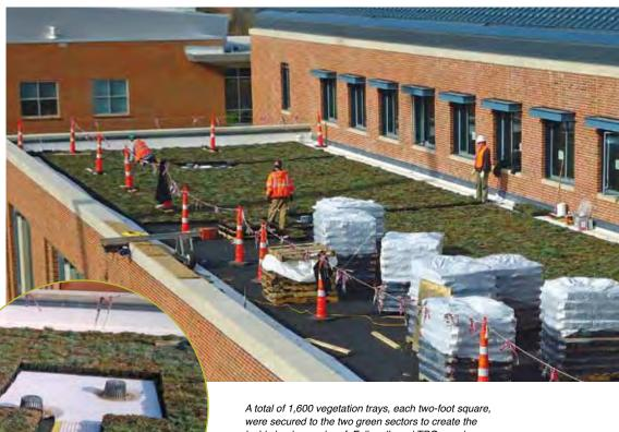
lushly landscaped roof. Fully adhered TPO membrane was applied to the entire roof, with tapered insulation affixed to the non-green sector.
