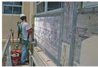
The scope of the 32 West Gore project increased significantly when Western discovered lath deterioration four inches deep—twice that originally anticipated. Swing-stage work requirements and ongoing tenant/guest access made safety a primary consideration. Both the finished project and Western process earned Orlando Health praise.
