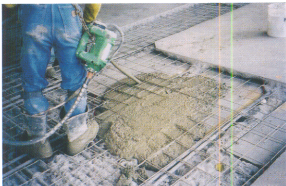
An asphalt overlay masked the degree of damage to the garage, which required over 15,000 sq. ft. of full depth concrete repairs.
