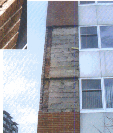
HSP reanchored the face brick using a plate-and-anchor system. Because the back-up block was only 4" deep, 6" x 6" metal plates were added to stabilize the walls.
