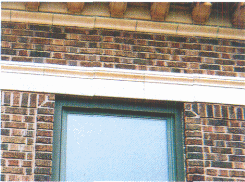
Cracked terra cotta pieces above windows were removed and replaced with cast stone replicas. The structural steel behind the masonry was repaired or replaced, and flashing was installed.
