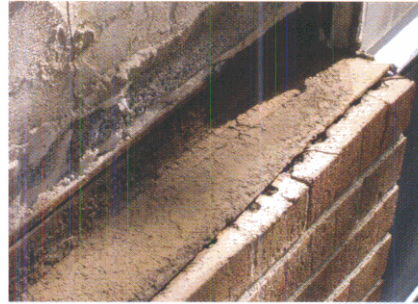
HSP reanchored the face brick using a plate-and-anchor system. Because the back-up block was only 4" deep, 6" x 6" metal plates were added to stabilize the walls.
