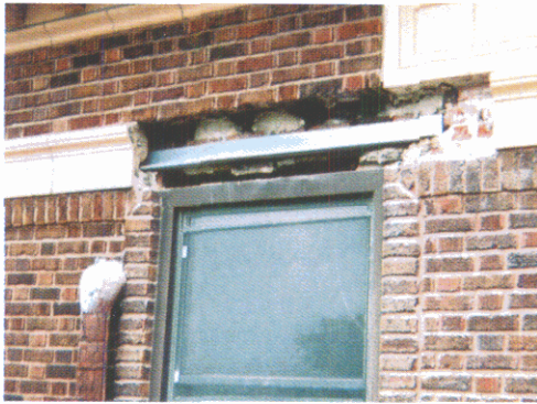
Cracked terra cotta pieces above windows were removed and replaced with cast stone replicas. The structural steel behind the masonry was repaired or replaced, and flashing was installed.
