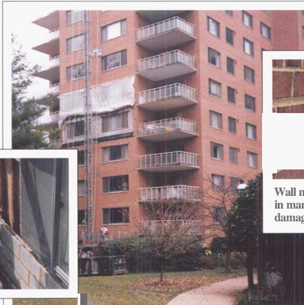
The Brisk crew removed displaced bricks, installed shelf angles and rebuilt damaged areas, using new brick that matched the original.
