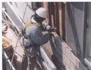
The Brisk crew removed displaced bricks, installed shelf angles and rebuilt damaged areas, using new brick that matched the original.
