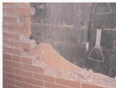
More than 1,200 new masonry veneer anchors were installed.
