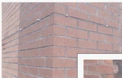
Western re-laid 15,000 bricks and cut new expansion joints on both buildings.
