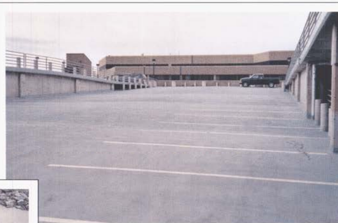
The Government Center Parking Terrace is a five-level, post-tensioned structure. Western kept a minimum of 75% of spaces available throughout repairs.
