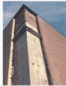
Western removed and replaced the old brick from two corners of the Neckers Building.
