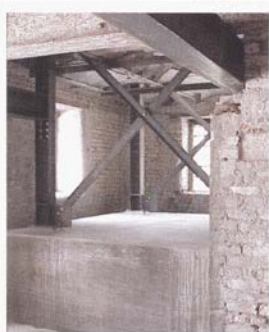
Upper: The masonry walls were in danger of collapsing, due to deterioration of the foundation. Above: Steel towers erected inside the structure stabilize the walls.
