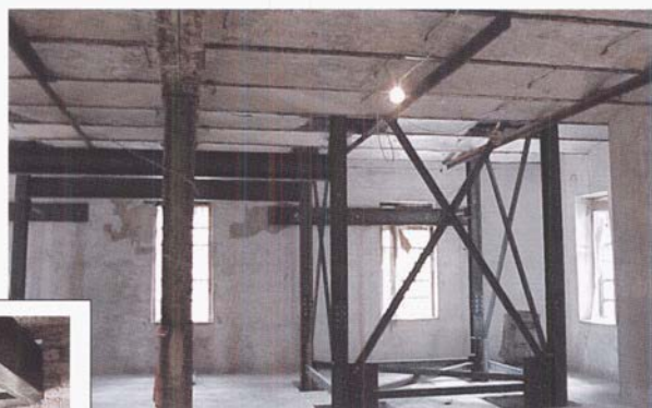
Upper: The masonry walls were in danger of collapsing, due to deterioration of the foundation. Above: Steel towers erected inside the structure stabilize the walls.
