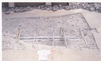
In addition to recoating the parking deck, the project also included concrete repair and patching.
