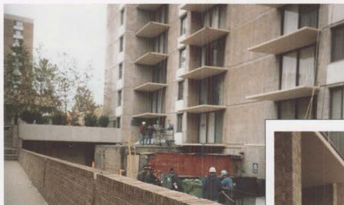
Railings were removed by hand and refitted with aluminum shoes and stainless steel hardware.
