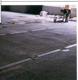
The repair solution involved inserting five T-stiffeners at each of the deck's 32 double-T joints.
