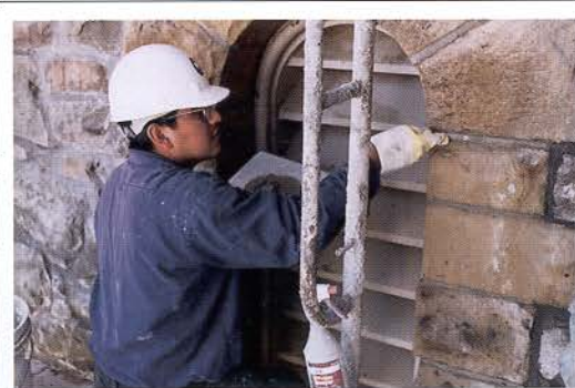
Crews repointed 100 percent of exterior surfaces.
