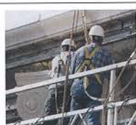
Some 1,200 fiberglass replacement panels were used in restoring 400 Royal.
