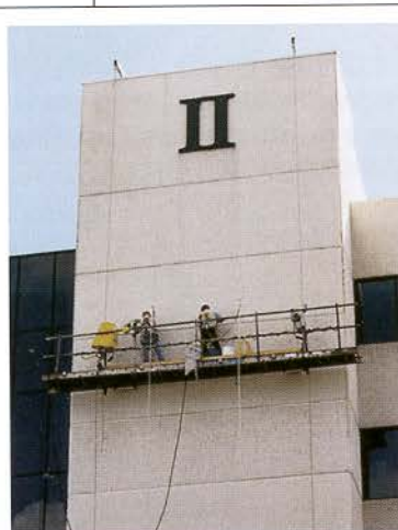
Routing and recaulking were added to the task-list when post-cleaning inspections revealed precast panel deterioration.
