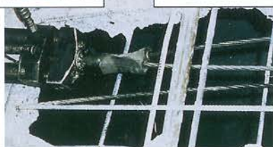
More than 400 of the garage's half-inch strand tendons required replacement or repair.
