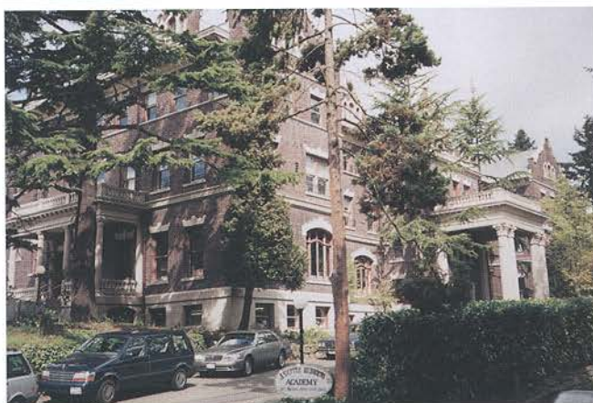
Matching the building's original materials—clinker-type brick, hand-molded concrete and terra cotta—proved a challenge well-met.
